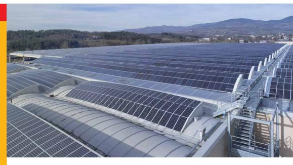
For this project, Baraclit b.POWER and Energy Resources, a leading company operating in the field of renewable energies, required the installation of photovoltaic modules on suitable shed roofing and flat roofing (pointing 12° south west) with a pitch of between 10° and 35° (according to the type of construction system) in order to ensure constant elevated exposure to the sun's rays for years to come.
